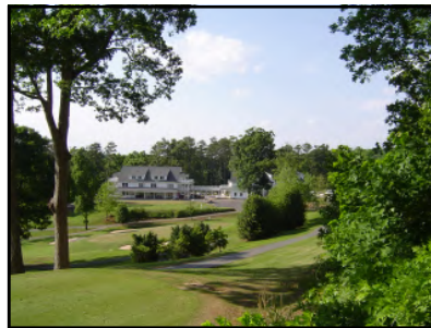
1913 Badin Inn from the hill above the historic building
